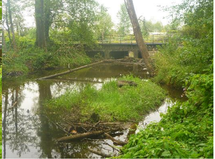
Photo 4 Downstream view towards railway bridge
