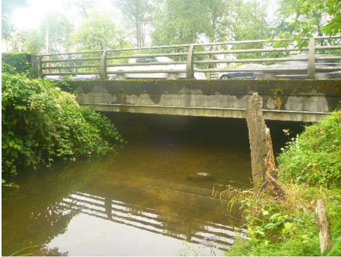
Photo 3 Downstream view towards 1 st St bridge
